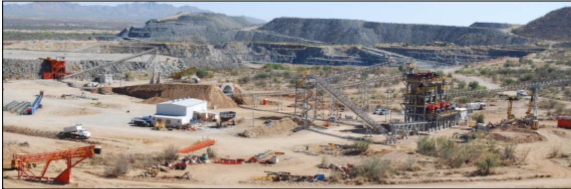
Brand new crushing system – 95% complete.
